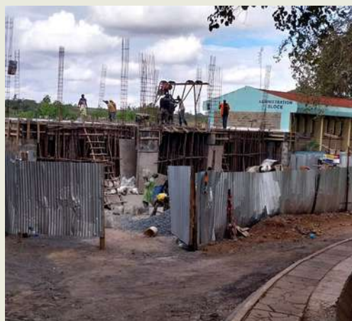
Construction of new office block
