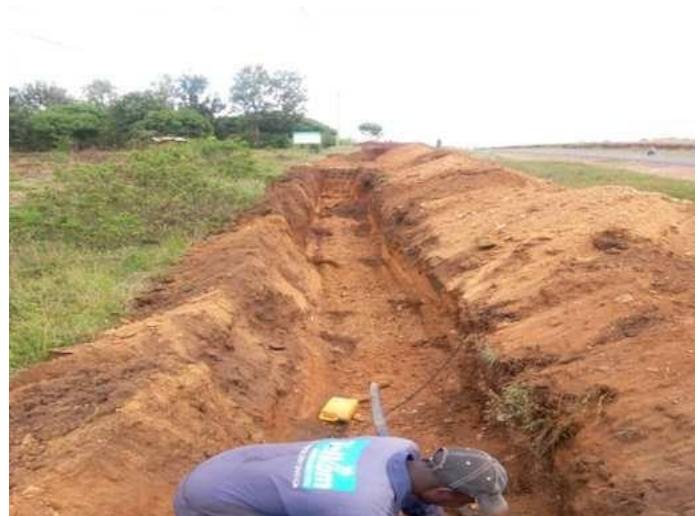
reinstatement of fiber cables
