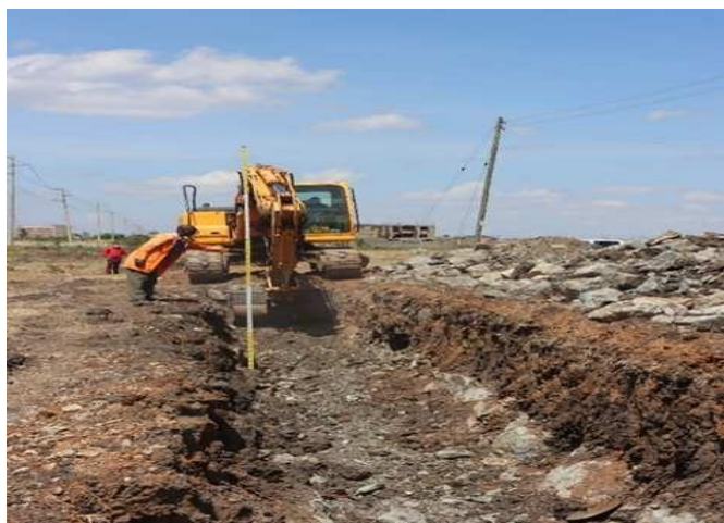
Excavation of diversion trench.
