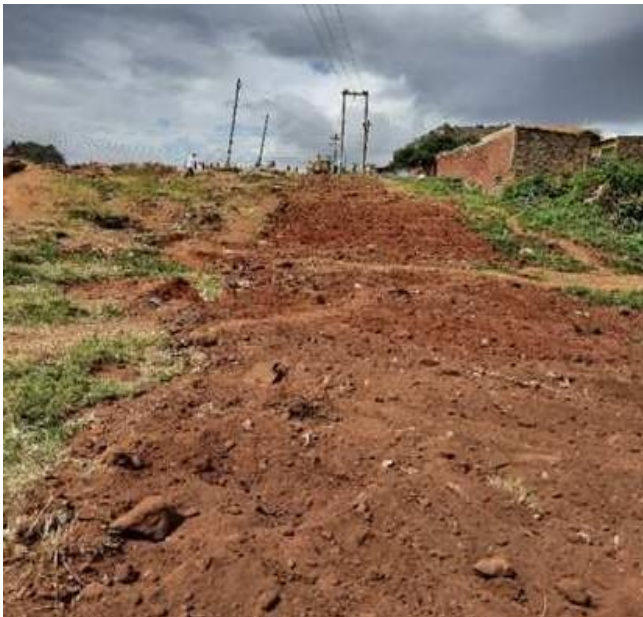
160mm Reinstatement to original ground level.
