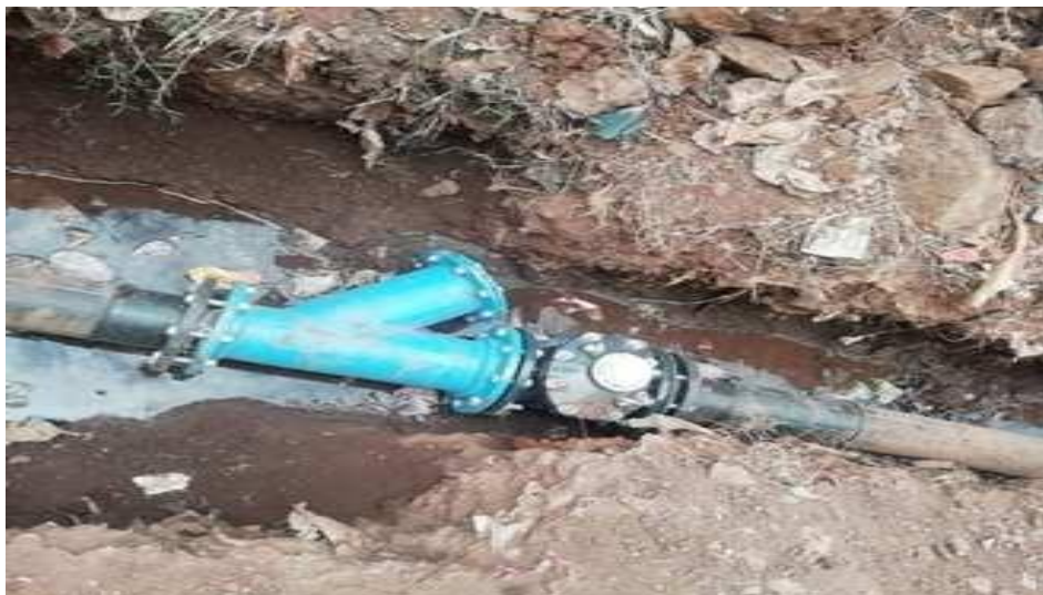
Installed meter and strainer.
