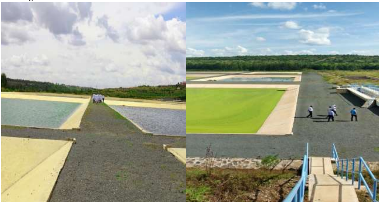
New sewerage ponds in series at Kang'oki sewerage treatment
